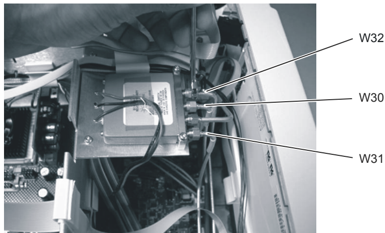
Figure 4-48. Removing the Cables from the Coaxial Switch
